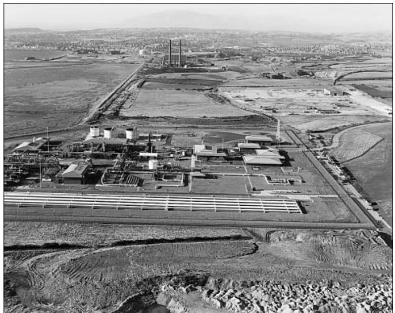
Fig. 2. View looking north showing the site bounded by the existing South Morecombe Terminal to the south and Roosecote power station to the north, with Barrow-in-Furness beyond
